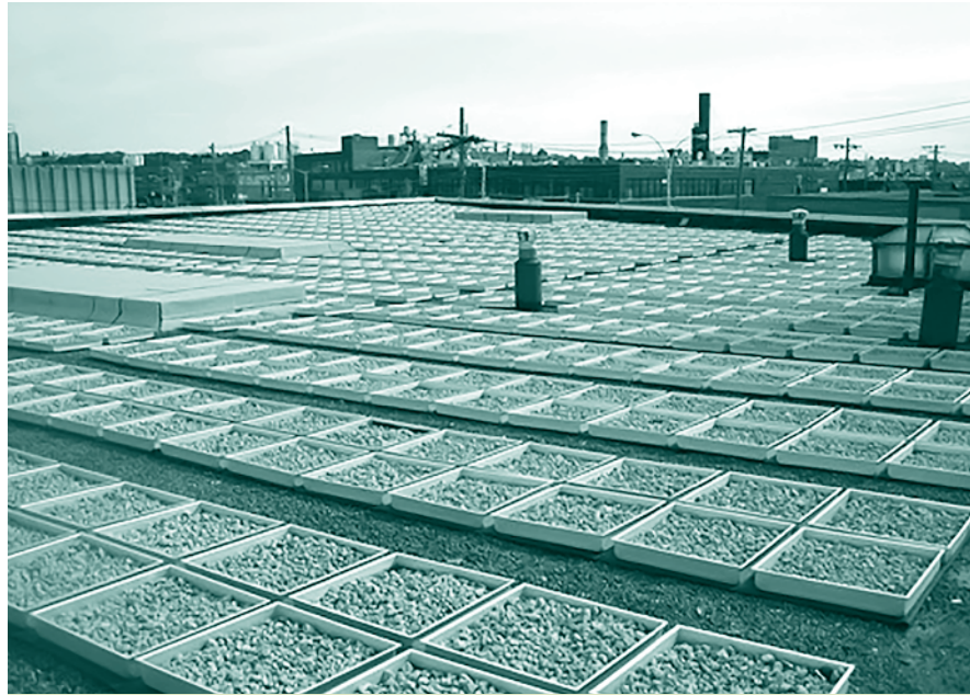
A water retention or “blue” roof in New York City. The roof is designed to temporarily retain water and gradually release it through weirs on roof drains.
